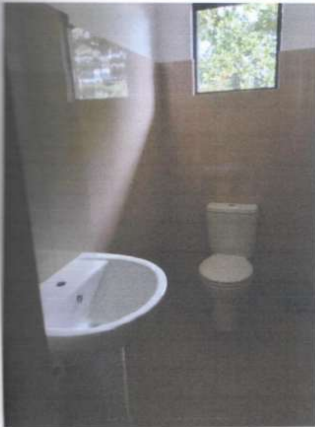
Bathroom fitting fixing on progress
