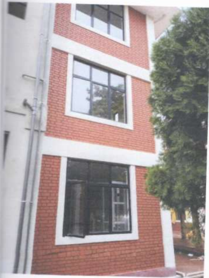
External painting on progress
