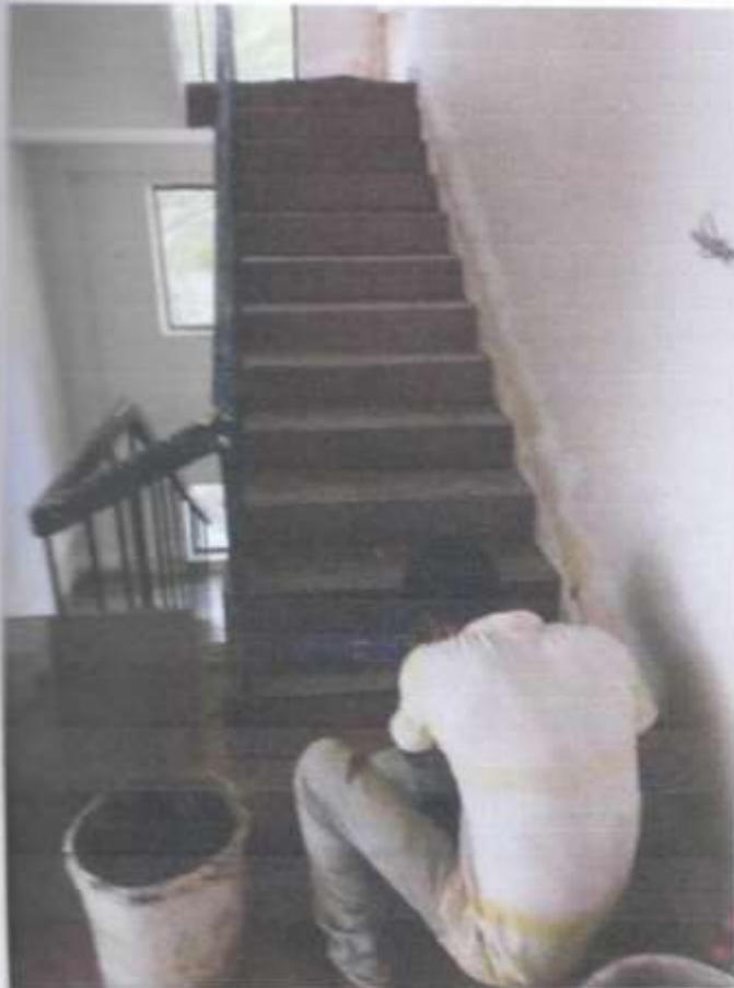
Staircase tiling work on progress
