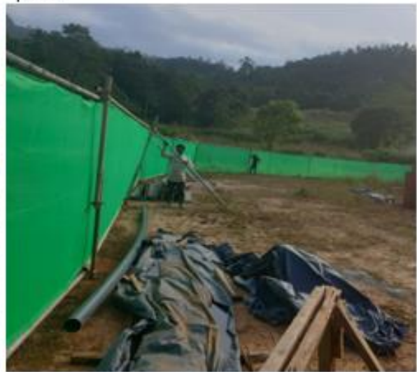
Galaha DHC: Noise/dust barriers erected around the site
