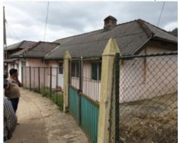
Nanu Oya MPCU: Construction has to be carried out next to a busy road
