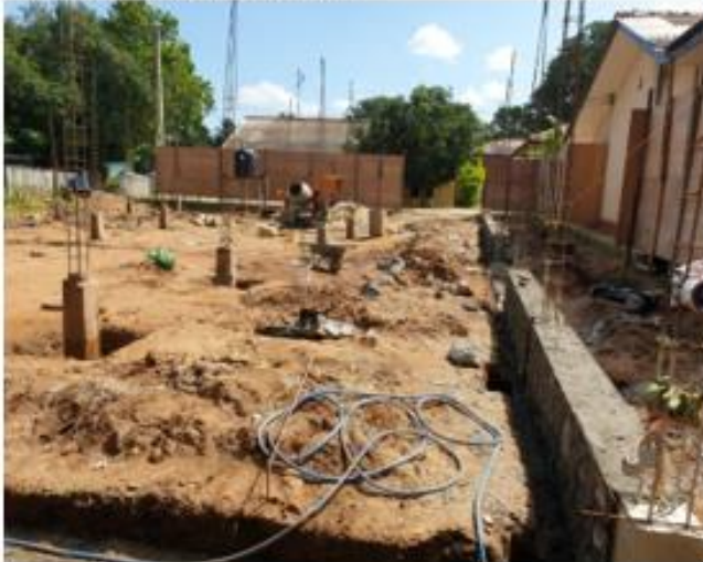
Thanamalwila DHB: The site has been separated by erecting noise/dust barriers
