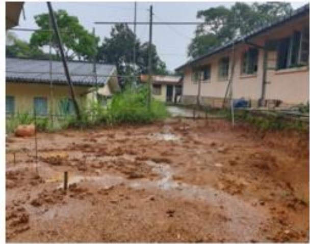
Laxapana DHC: Construction has to be carried out with minimum disturbance to the hospital
