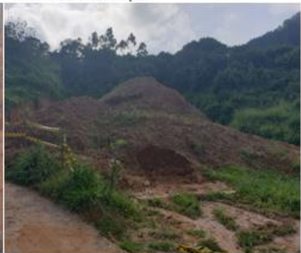
Dolosbage DHC: Excavated soil being stored at site without cover and obstructing drainage paths
