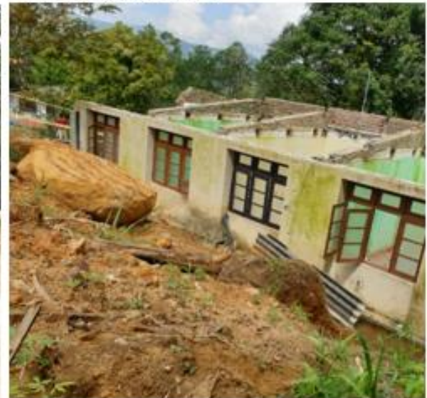
Pundalu Oya: Slopes that need stabilization prior to construction of the new building
