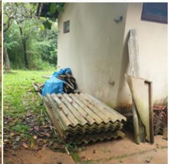
Damminna PMCU: AC sheets improperly stored at site
