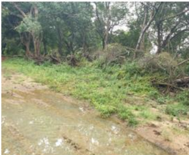
Ellewewa PMCU: Trees felled are lying within the site; water puddles within the site
