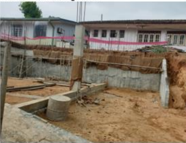
Meegahakiula DHB: Slopes being strengthened by constructing retaining walls
