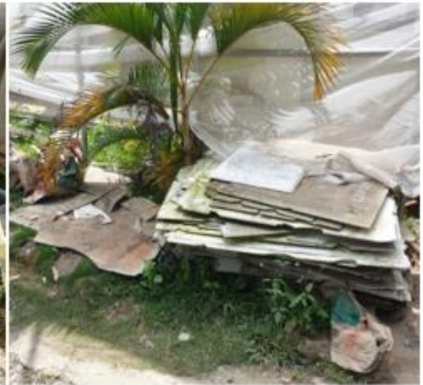
Pundalu Oya PMCU: AC Sheets stacks in the site in an unsafe manner
