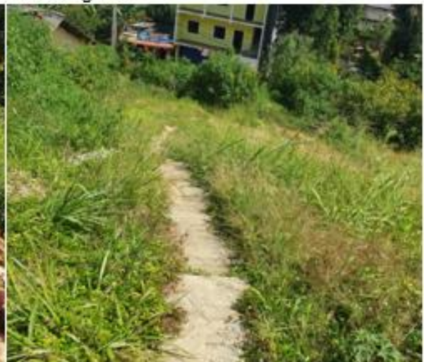
Madulkele DHB: There is no proper access road to the site
