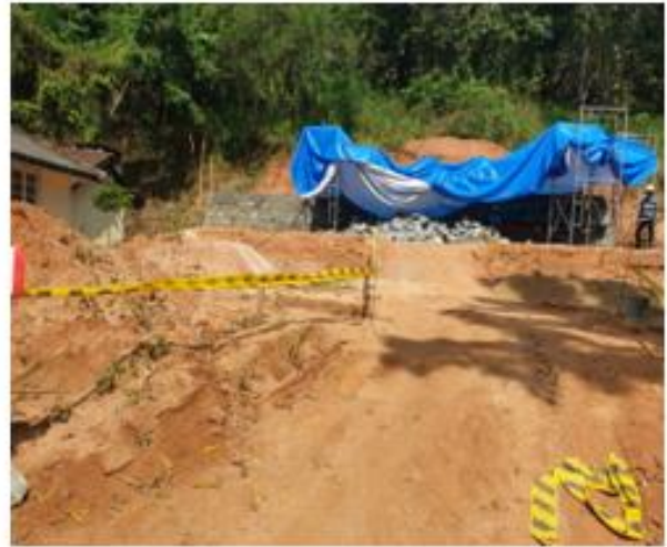
Hataraliyedda DHC: Proper retaining wall being constructed under shade provided for laborers
