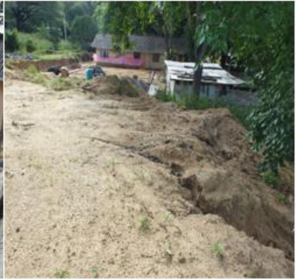
Dombagahawela PMCU: Excavated soil needs to be levelled in the backyard of the hospital.
