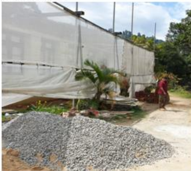
Pundalu Oya PMCU: Dust barriers erected around the site
