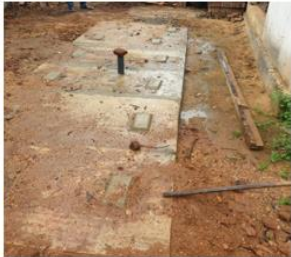
Galenbindunuwewa DHB: Properly sized septic tanks/soakage pits being constructed
