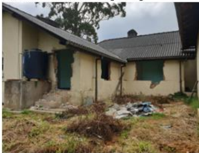
Nanu Oya PMCU: Demolition of the existing building being carried out
