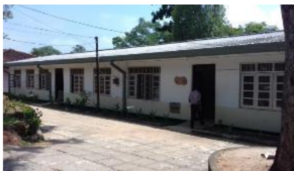
Some images of PHC facilities in the current package using AC sheets (Hambegama DH, Ettampitiya DH, and Meegahakiwula DH)
